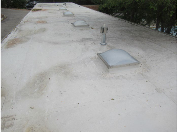
Thermoplastic roof at lodge building
