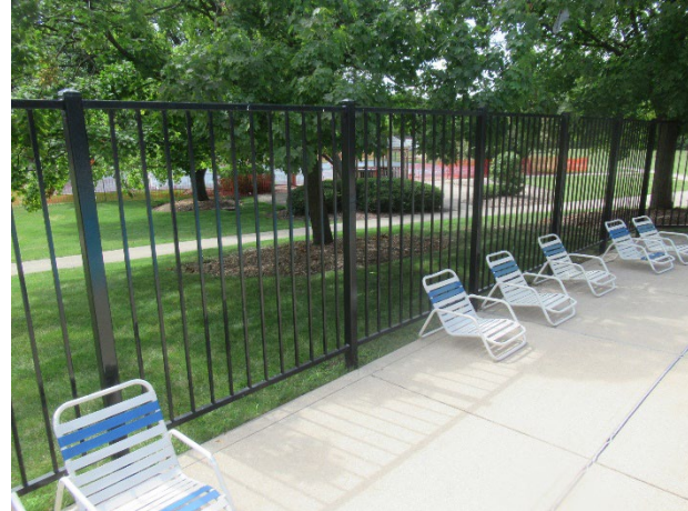
Aluminum picket fence at towers pool
