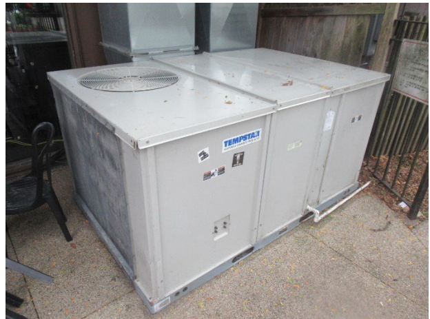
Rooftop heating and cooling unit (7.5-ton)
