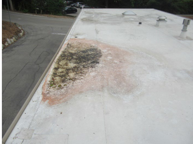
Evidence of water ponding at lodge roof
