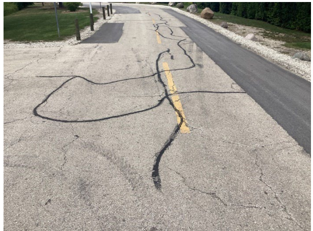
Cracks and previous repairs throughout section of street to be repaved
