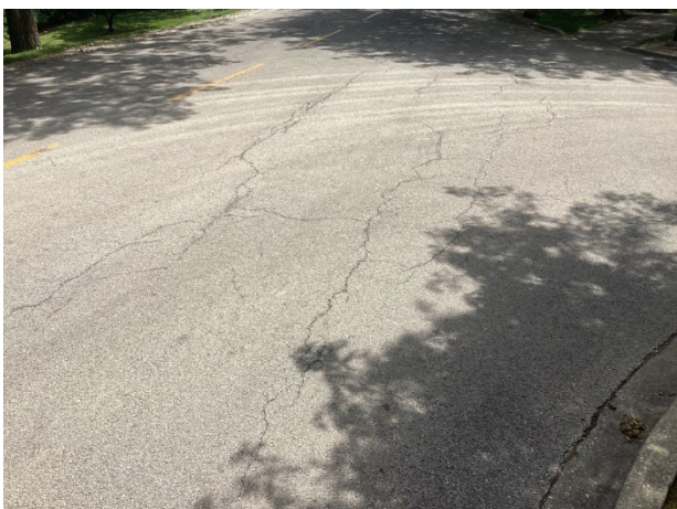
Unrepaired cracks at street intersection
