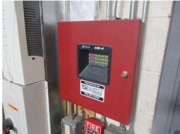
Maintenance shop life safety system panel
