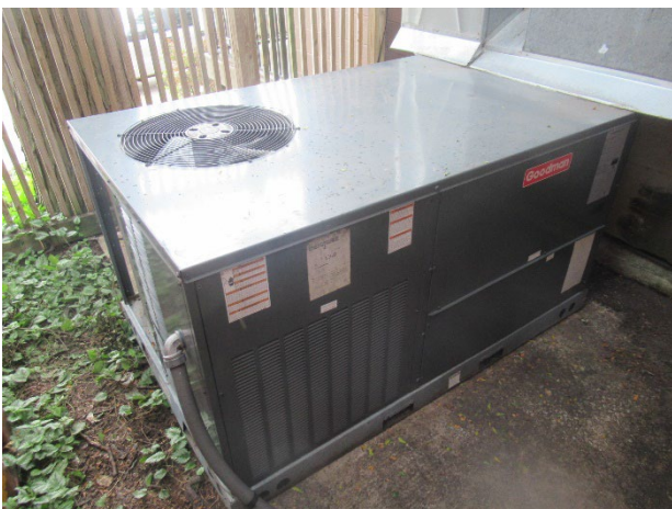
Rooftop heating and cooling unit (5-ton)
