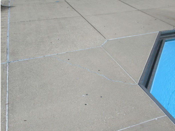
Repaired cracks at towers pool deck
