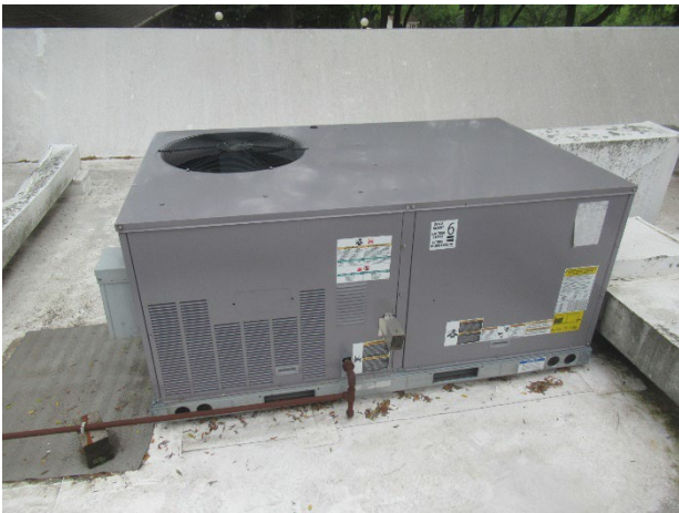
Rooftop heating and cooling unit (4-ton)
