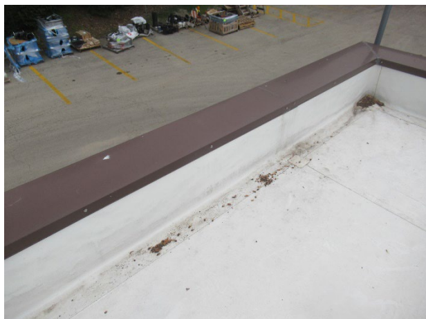
Parapet wall and cap in good condition
