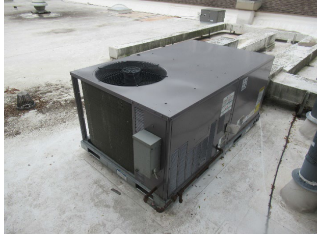
Rooftop heating and cooling unit (6-ton)
