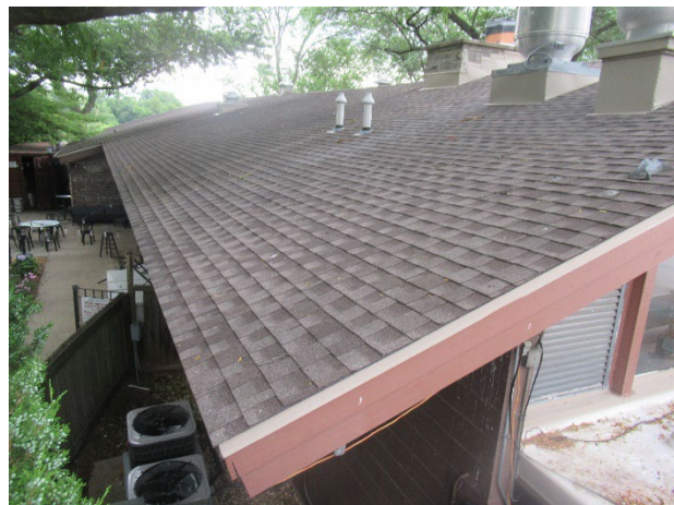
Lodge sloped roof system and penetrations
