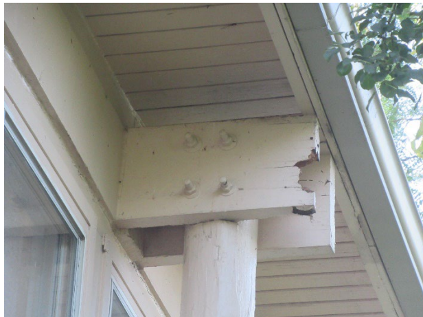
Wood deterioration at office exterior
