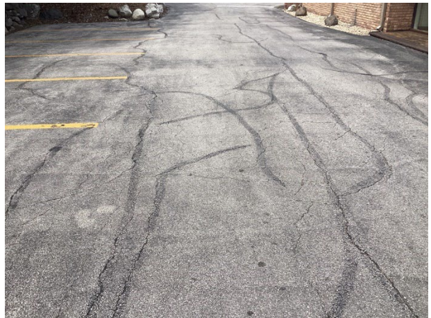
Cracks and previous repairs at lodge parking area
