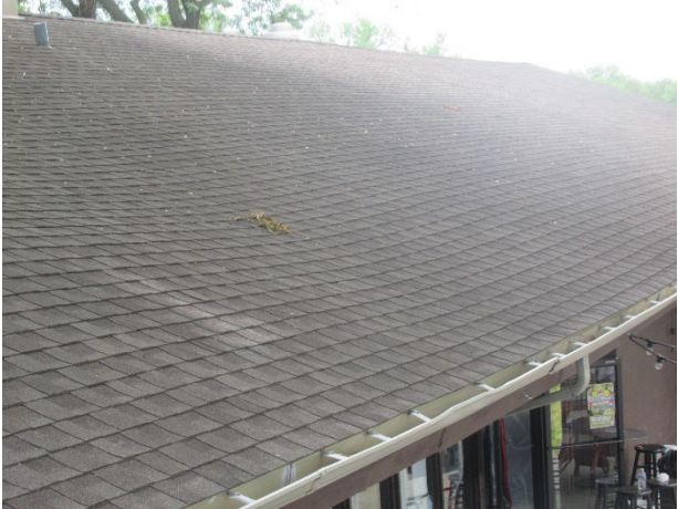
Sheathing deflection at east section of lodge roof
