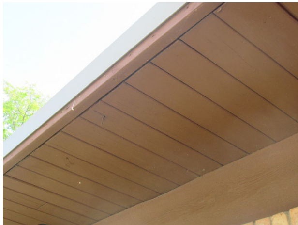
Wood soffit and fascia at lodge exterior
