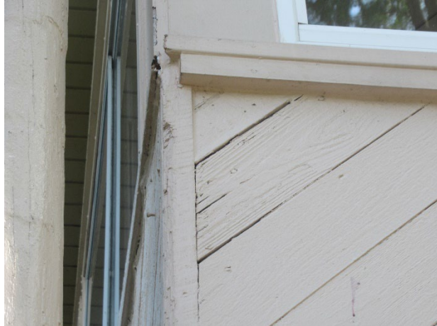
Siding cracks and delamination
