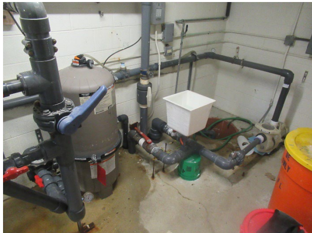
Pool pumps and filter
