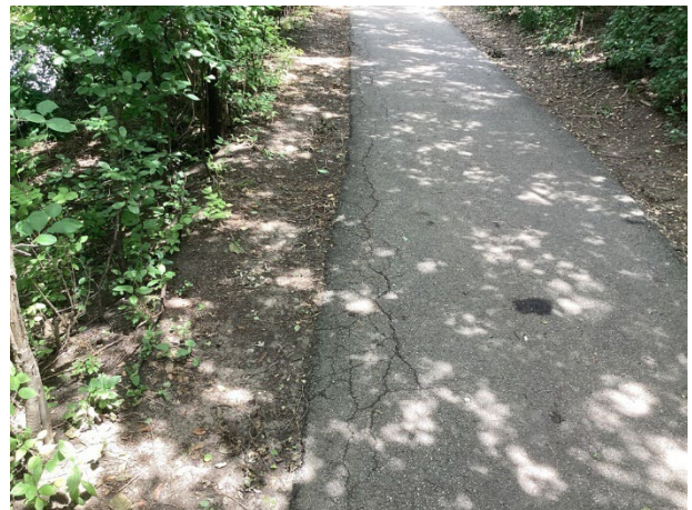
Cracks at walking path edge
