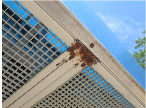
Rust at metal awning frame
