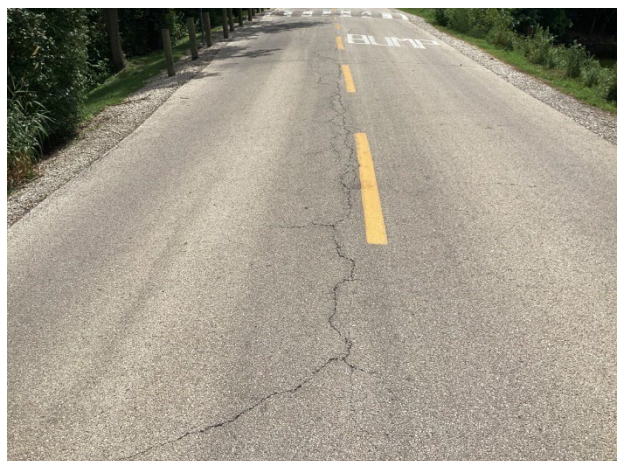
Unrepaired centerline cracks
