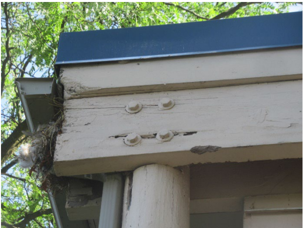
Wood deterioration at office exterior
