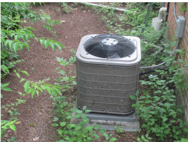
Laundry building condensing unit
