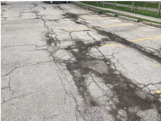
Pavement failure at lodge parking area
