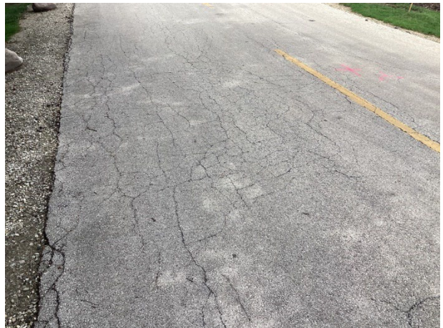
Pavement settlement and alligator cracks
