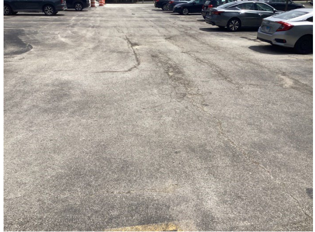
Centerline deterioration at parking area drive lane
