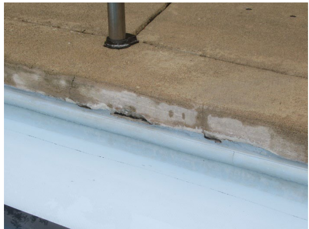
Cracks and deterioration at the office pool deck coping
