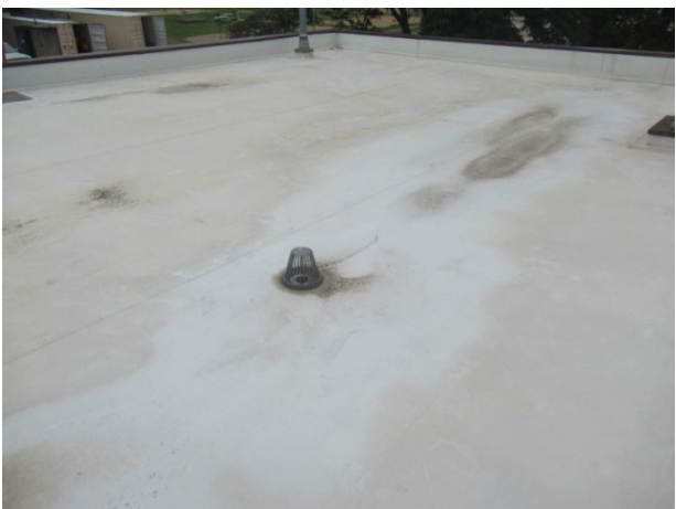
Minor deflection at maintenance building roof
