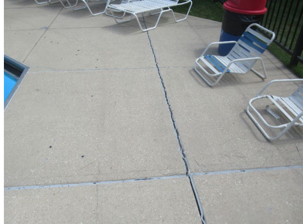
Control joint sealant deterioration at towers pool deck
