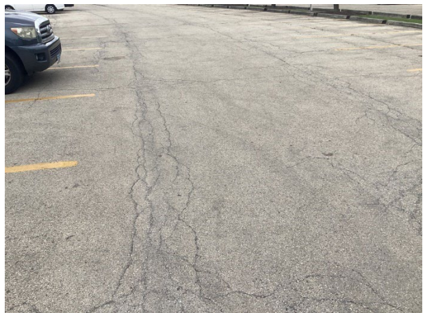
Unrepaired cracks and settlement
