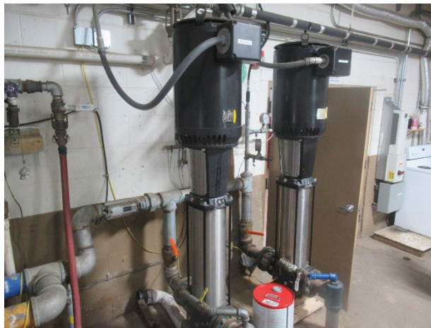
60-HP pumps to circulate snow making system water
