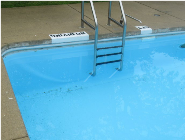
Loose vinyl liner at office pool wall
