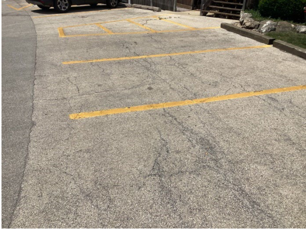
Example of parking area with cracks throughout
