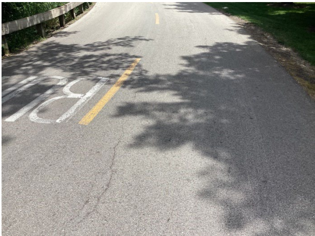
Isolated and minor cracks
