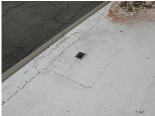
Roof drain missing cover
