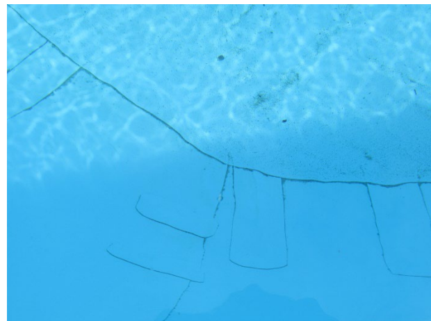
Vinyl liner repairs
