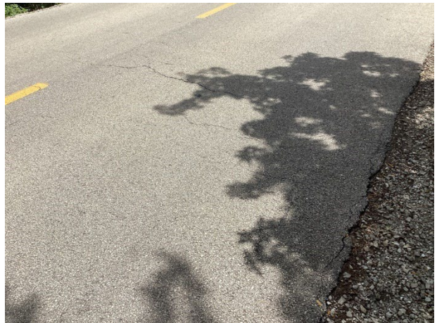
Isolated and minor cracks
