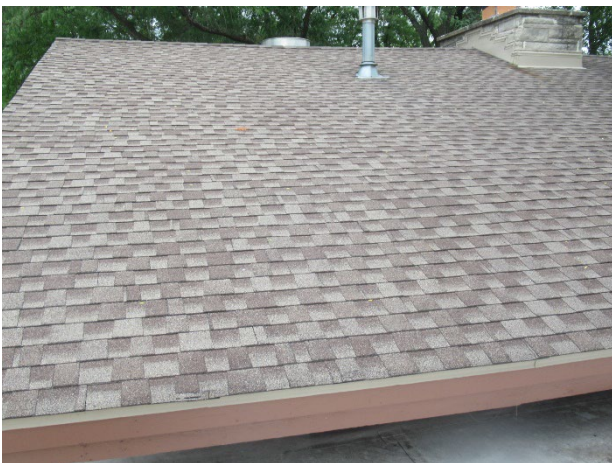
Laminate asphalt shingle roof assembly at lodge
