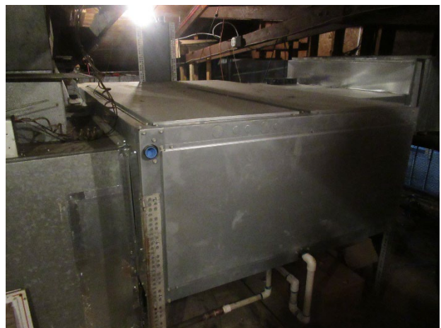
Lodge attic air handling unit (replace parts as necessary using funds from operating)
