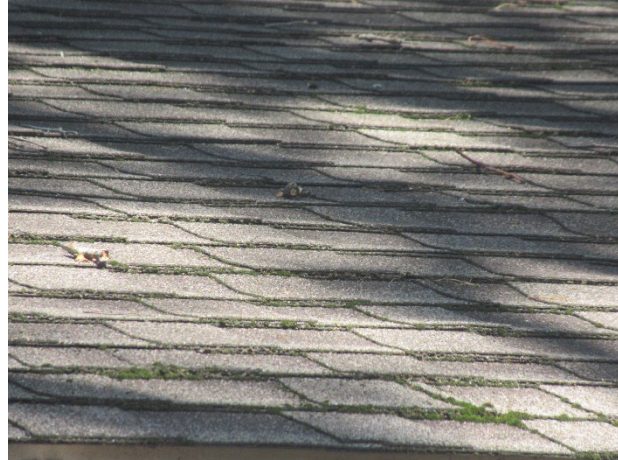
Weathered shingles and organic growth
