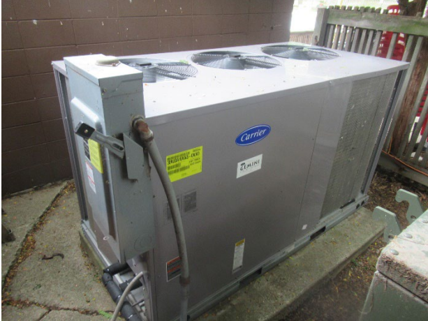
Rooftop heating and cooling unit (15-ton)
