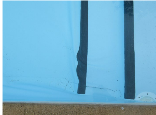
Vinyl liner repairs
