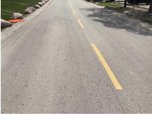
Crowned asphalt street pavement
